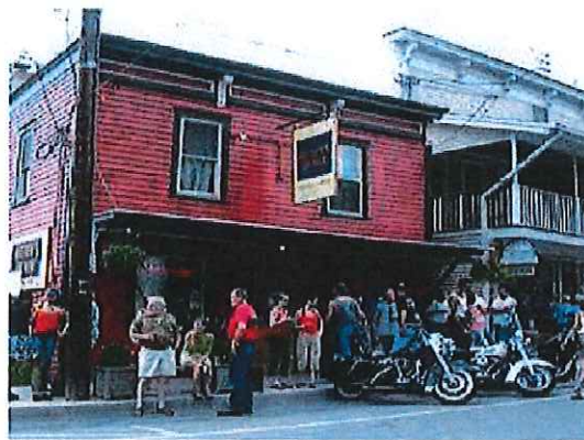
Blade sign projecting from upper story.
