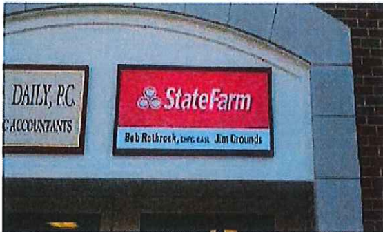
Wall sign located in sign band.
