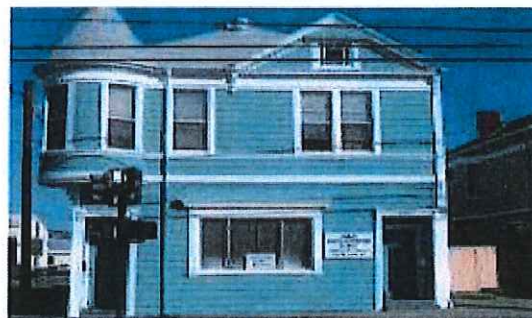
Wall sign on mixed use building.
