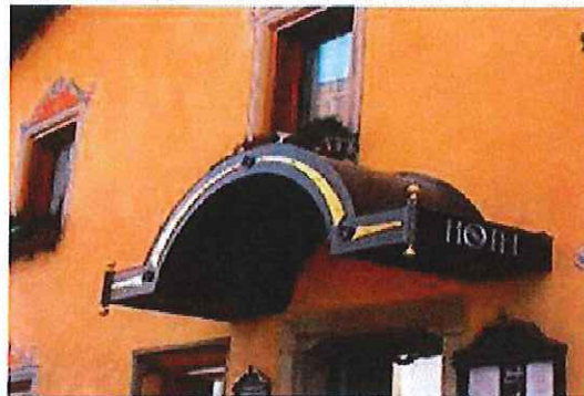
Sign on side of ornate canopy.
