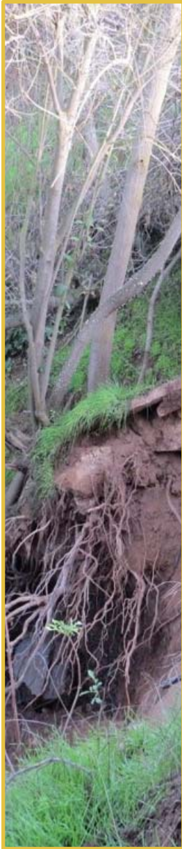
Seventh Street Storm Drain Repairs
