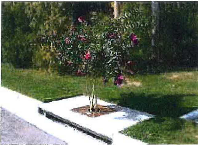
Filterra® Stormwater Bioretention Filtration System
