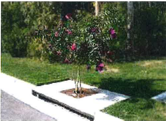
Filterra® Stormwater Bioretention Filtration System
