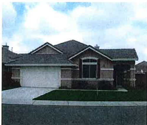
Discourage homes with recessed entry that limit the view of the street.
