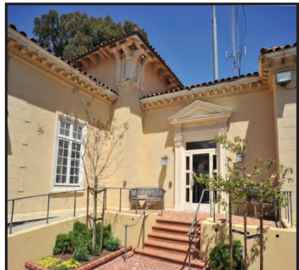
POLICE BUILDING ENTRANCE
