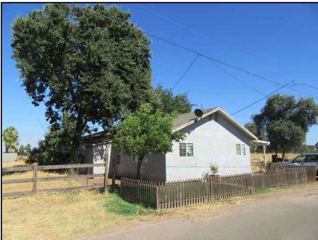
Existing home and outbuildings in the northwest corner of the site, looking southeast; 07/14/17.
