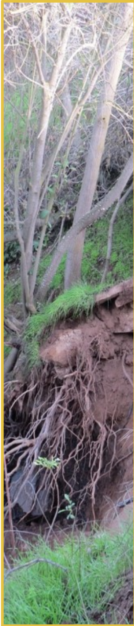
Seventh Street Storm Drain Repairs
