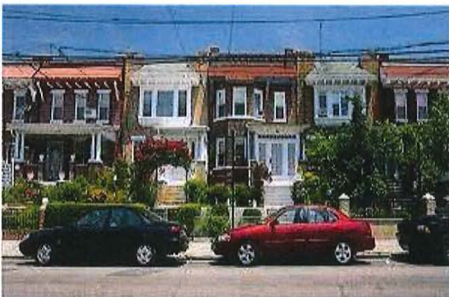
Row houses with terraced private yards
