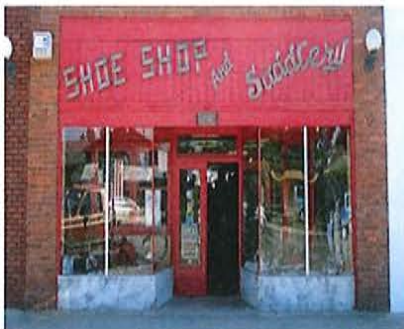
Shopfront windows and recessed along Santa Fe Street.
