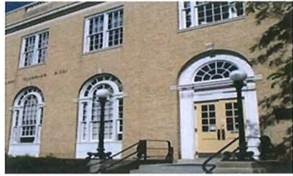
Framed formal entry, classical detailing.
