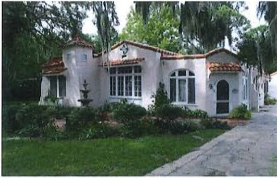
Roof treated with red tile.
