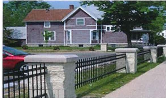
Masonry piers, caps, and ironwork.
