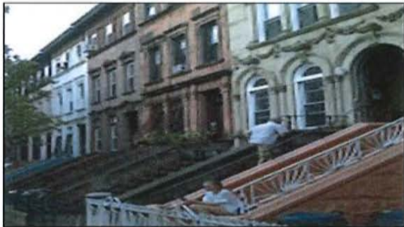
Stoop and recessed alcove provide entry to multiplex.
