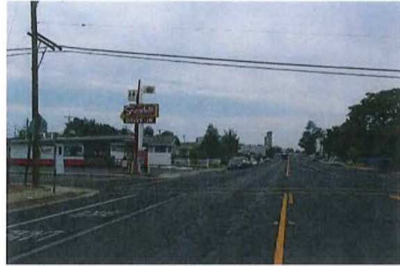
Atchison Street east of Third Street.
