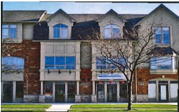
Base treatment, variation in materials, and unique roof forms create visual interest.
