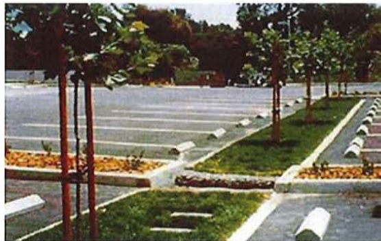
Bioswale water detention system internal to parking lot.
