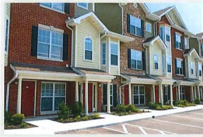
Single and multifamily bldgs.
