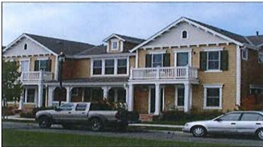
Roof overhangs and use of brackets support residential design.
