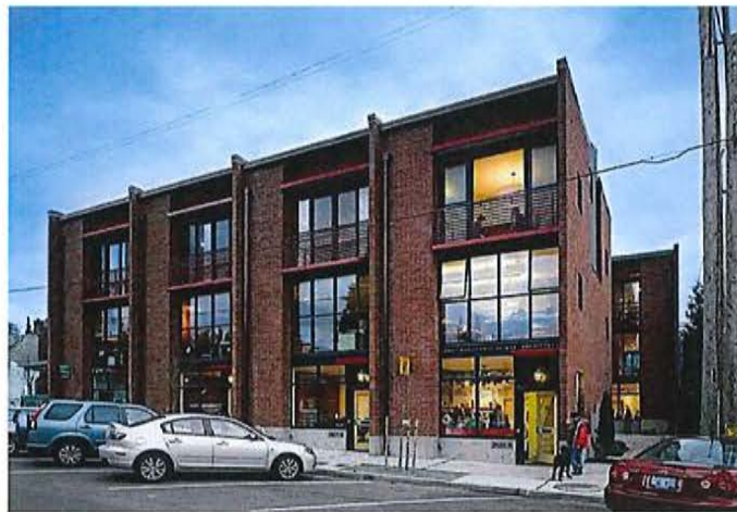
Adaptive re-use to live-work.
