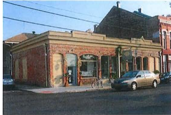
Single story building with brick and masonry facades.
