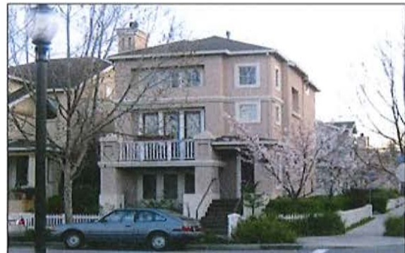
Recessed entry, balcony, belt courses and overhanging eave articulate building height.
