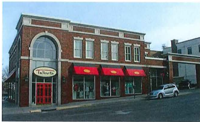
Parking located to rear.
