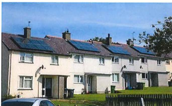
Row houses along a court.
