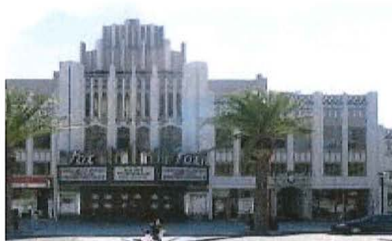
Distinctive columns separate individual shopfronts and often break the roof plane
