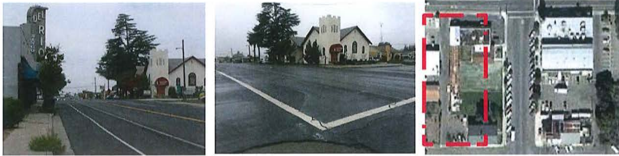
Existing conditions: Intersection of Atchison Street and Third Street.
