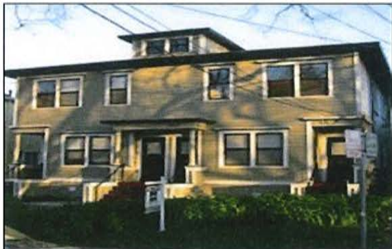
Shared stoop and porch on multiplex
