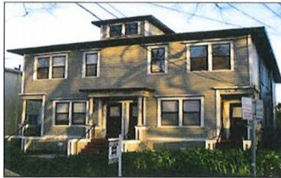
Light weight siding and earth tones support the community's vision for downtown.
