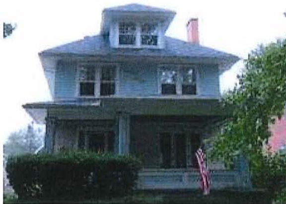
Double-hung windows and overhanging eaves.
