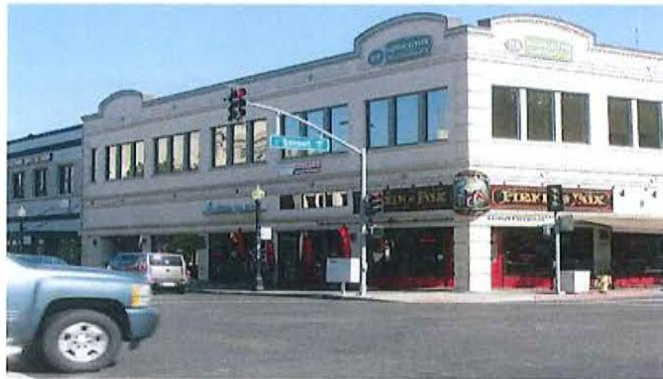
Offices over shop fronts
