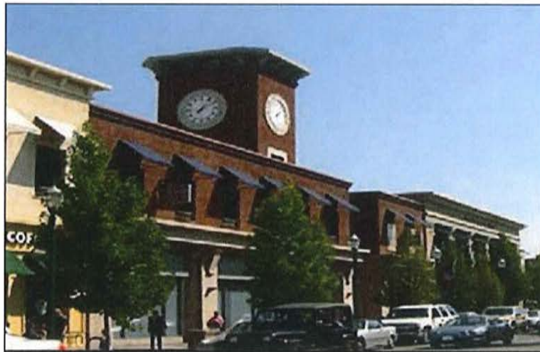
Offsetting of building bays and change in materials help to articulate this parking structure.
