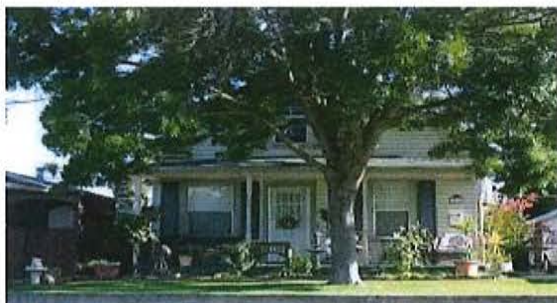
Near the corner of Third and Santa-Fe St. in the
