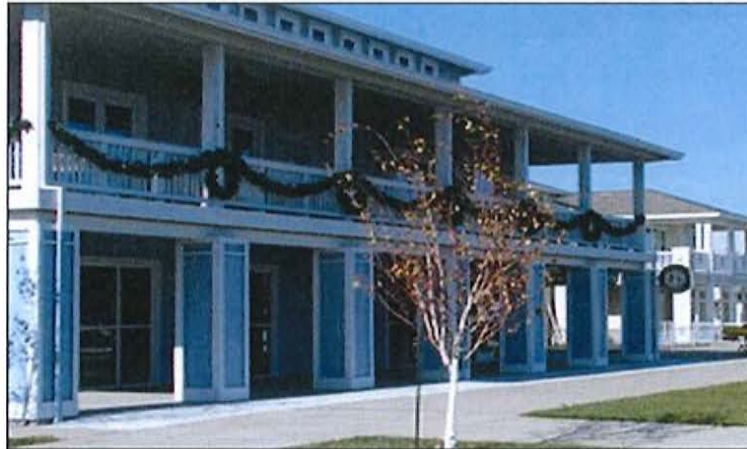
Arcade with terrace above
