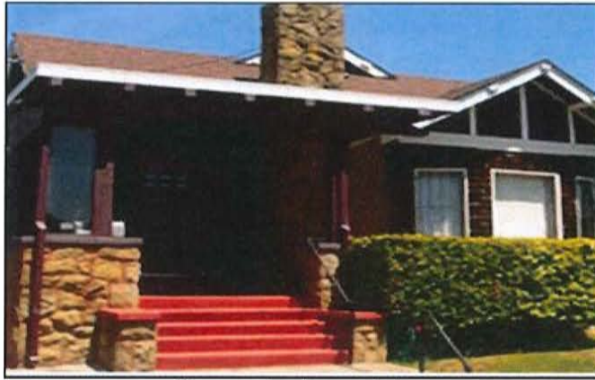
Recessed entry and stoop.
