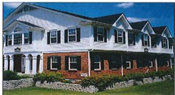
Multiplex with common yard.
