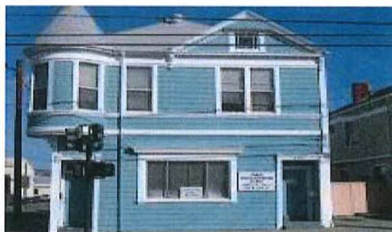
Wall sign on mixed use building.
