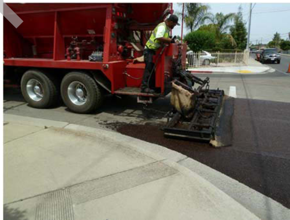
Slurry Seal Project - Funded by LTF
