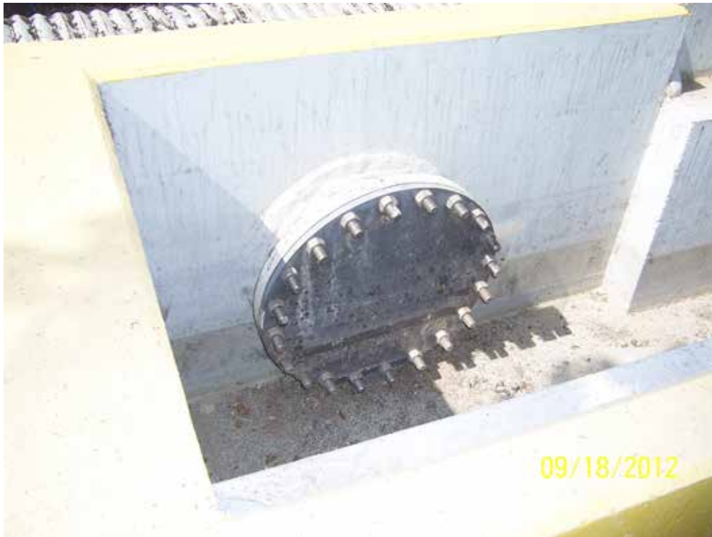
WWTP HEADWORKS BEFORE
