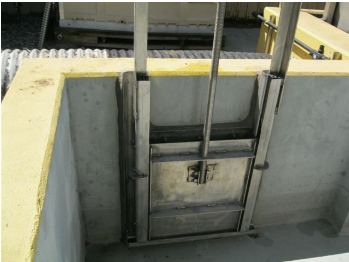
WWTP HEADWORKS AFTER
