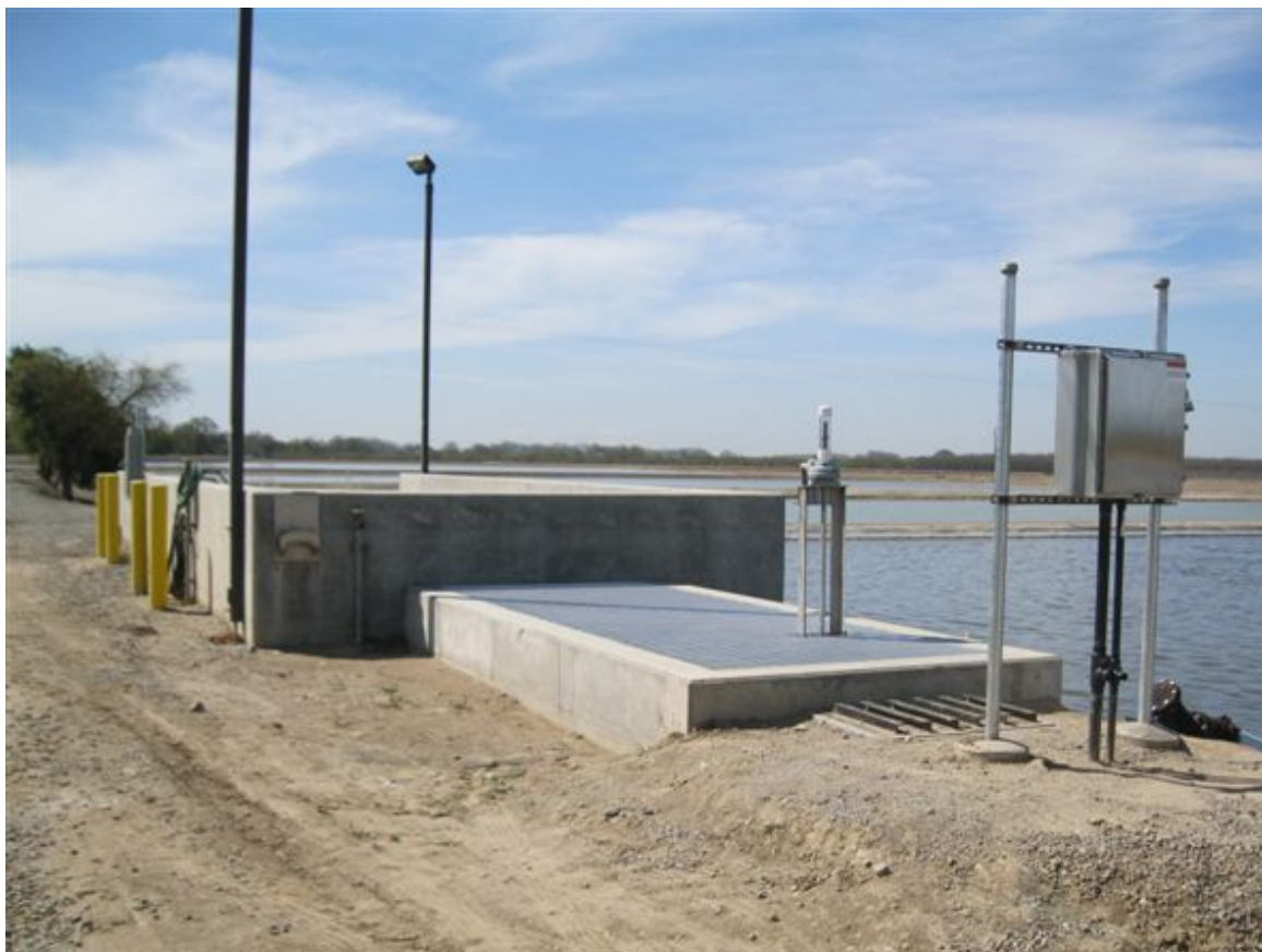
VACTOR DUMP STATION AFTER
