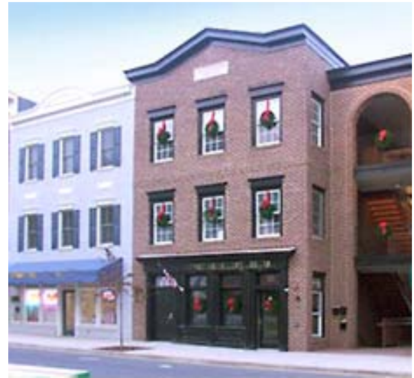
Figure LAND-2. Mixed Use Development. Housing above commercial, or “vertical mixed-use,” is encouraged within the Mixed Use (MU) Land Use Designation.
