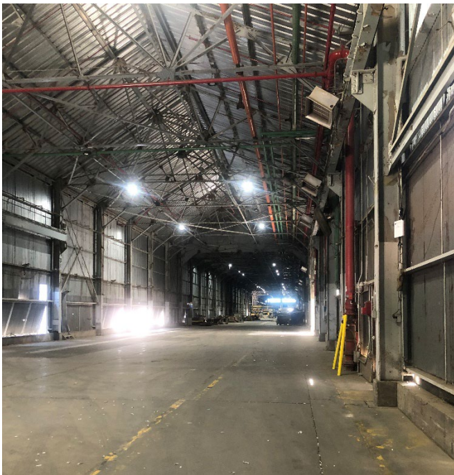
Building 1 – View toward East 16 SEPTEMBER 2025
