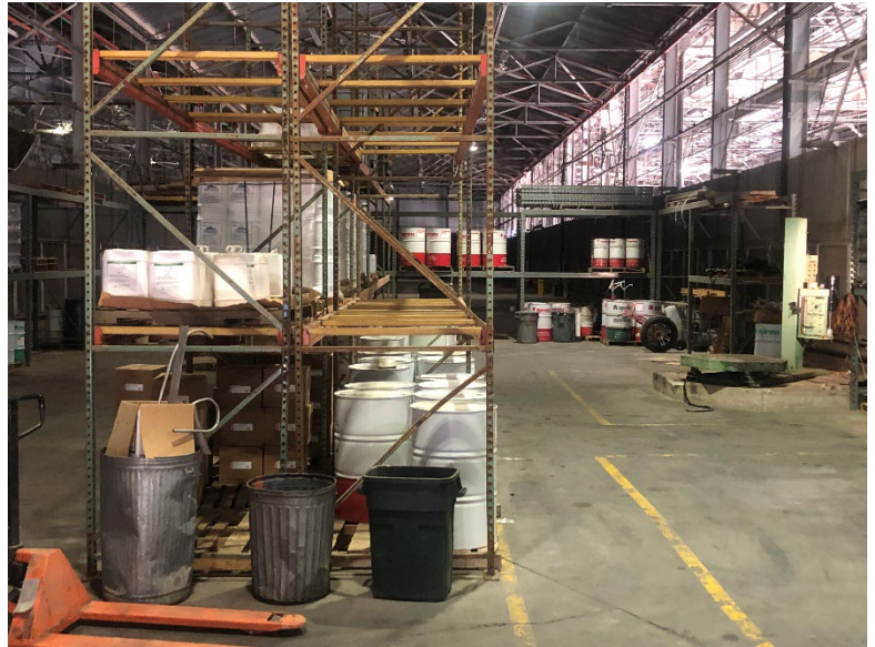
Bldg. 160 Between Bldgs. 2 & 3 – View toward East 16 SEPTEMBER 2025
