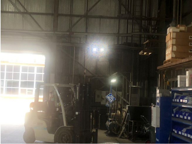
Bldg. 15 – View toward East 17 SEPTEMBER 2025
