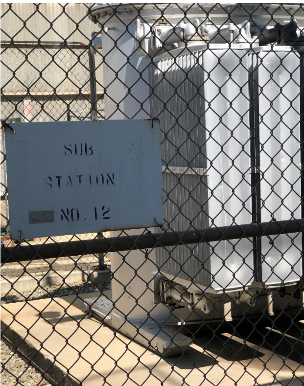
Substation 12 – View toward Northeast 17 SEPTEMBER 2025
