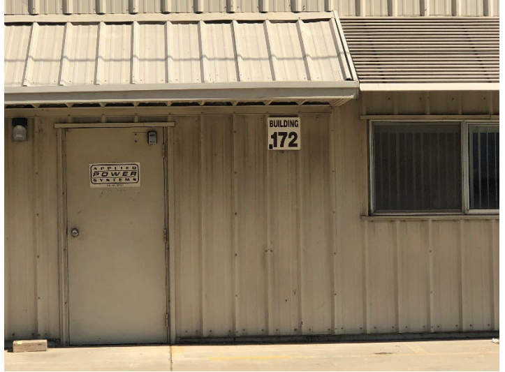
Bldg. 172 – View toward East 16 SEPTEMBER 2025
