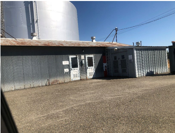
Bldg. 137 – View toward Southeast 16 SEPTEMBER 2025
