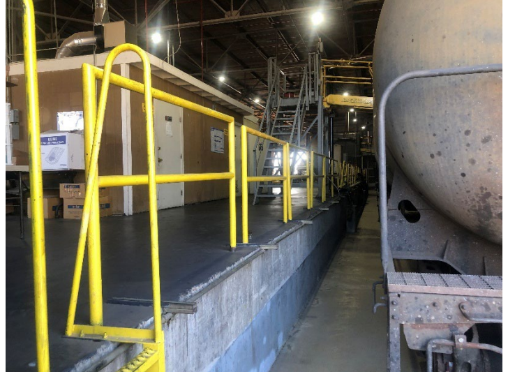
Bldg. 11 – View toward South 16 SEPTEMBER 2025
