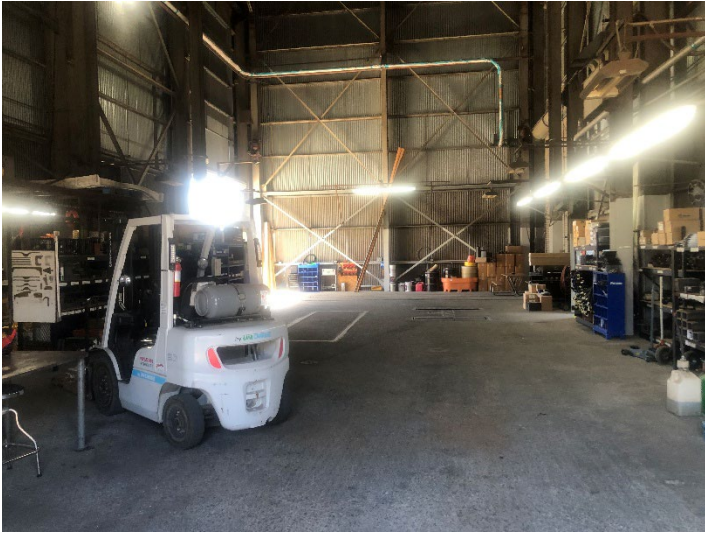
Bldg. 15 – View toward West 17 SEPTEMBER 2025
