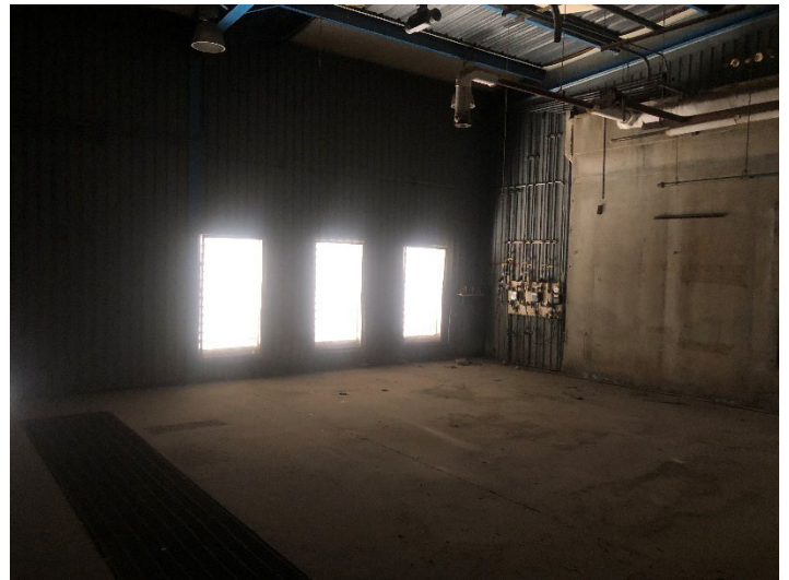
Bldg. 156 – View toward Southwest 16 SEPTEMBER 2025
