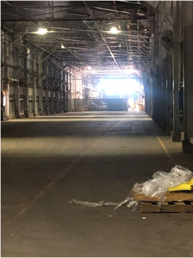
Building 2 – View toward East 16 SEPTEMBER 2025
