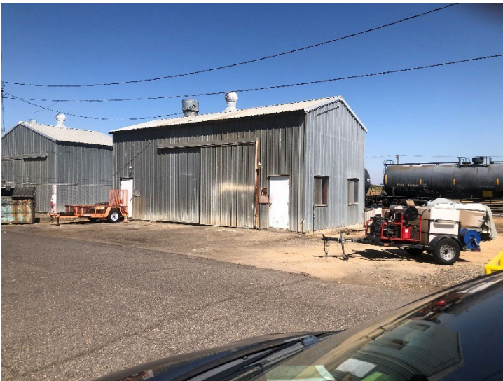
Bldg. 169 – View toward Northeast 16 SEPTEMBER 2025
