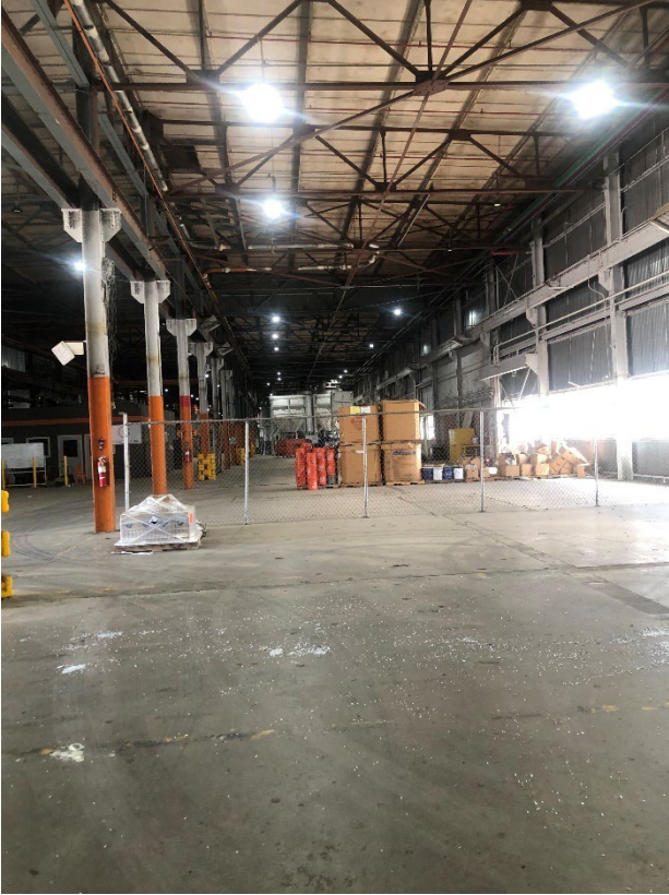
Building 7 – View toward East 16 SEPTEMBER 2025
