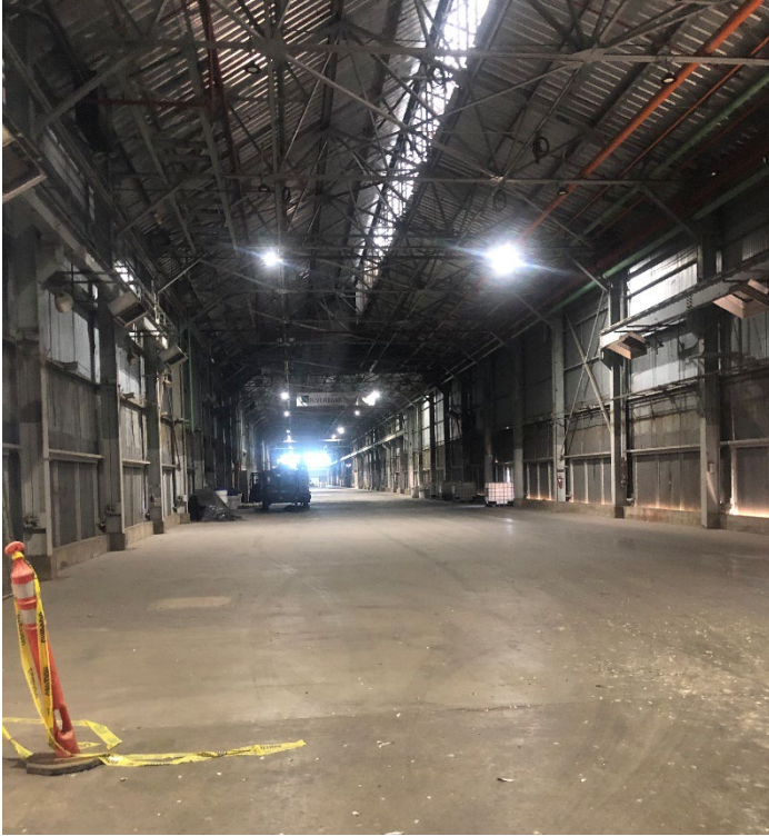
Bldg. 6 – View toward East 16 SEPTEMBER 2025
