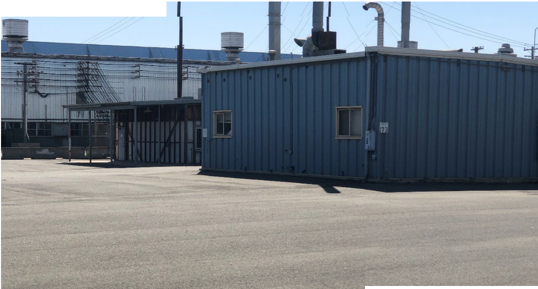
Bldgs. 43 & 173 – View toward Southwest 16 SEPTEMBER 2025
