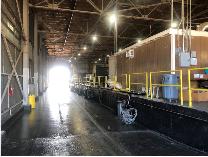
Bldg. 11 – View toward South 16 SEPTEMBER 2025
