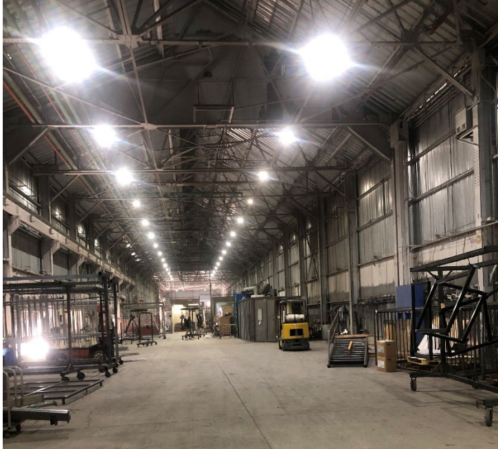
Bldg. 5 – View toward West 16 SEPTEMBER 2025
