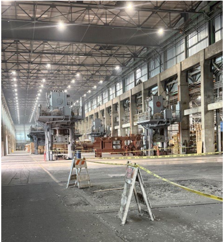
Bldg. 8 – View toward South 18 SEPTEMBER 2025
